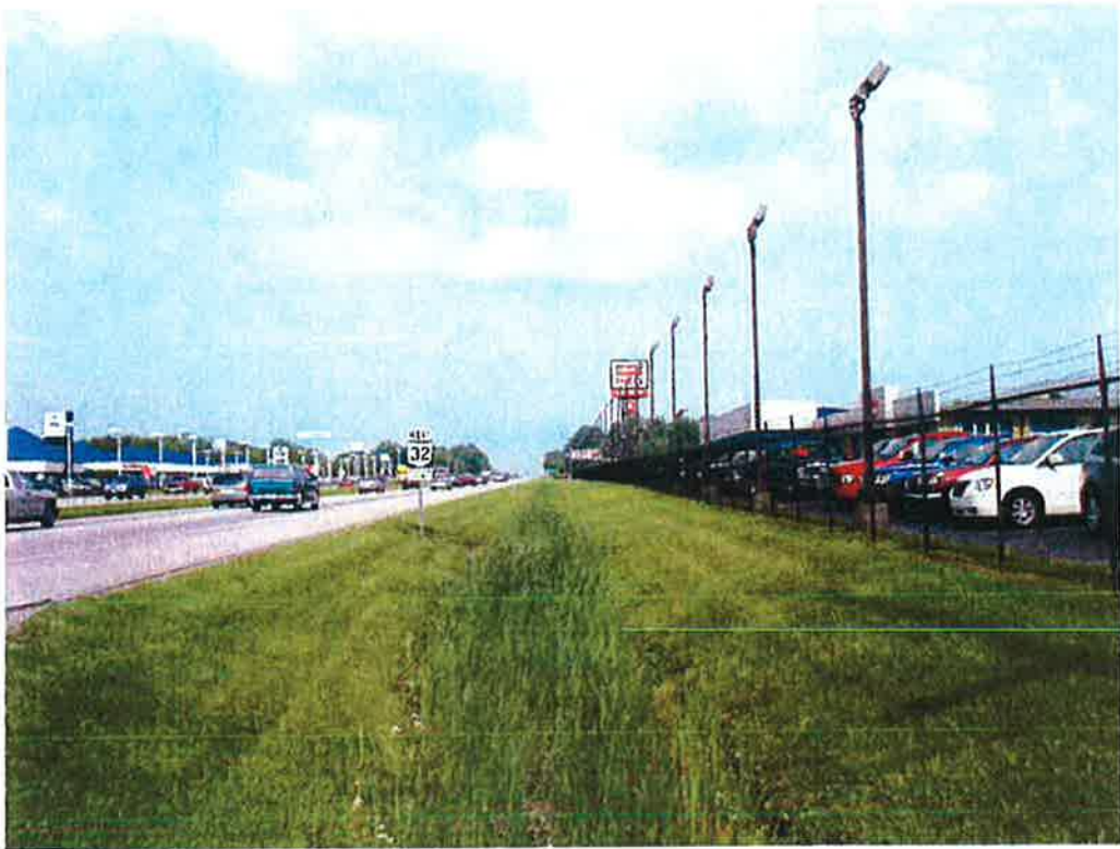
Looking west along north side of SR 32 from Elick Lane
