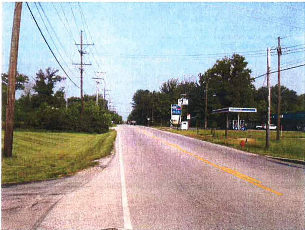
Looking west along Old SR 74 from Schoolhouse Road
